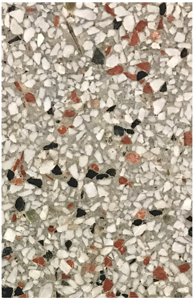
MEETING ROOM/DANCE HALL (16) & GENERAL AREAS (1, 2, 5B, 5C, 5D, 6, 7, 13, 15, 18, 19, 19A) EXISTING TERRAZZO- NEW TO MATCH
