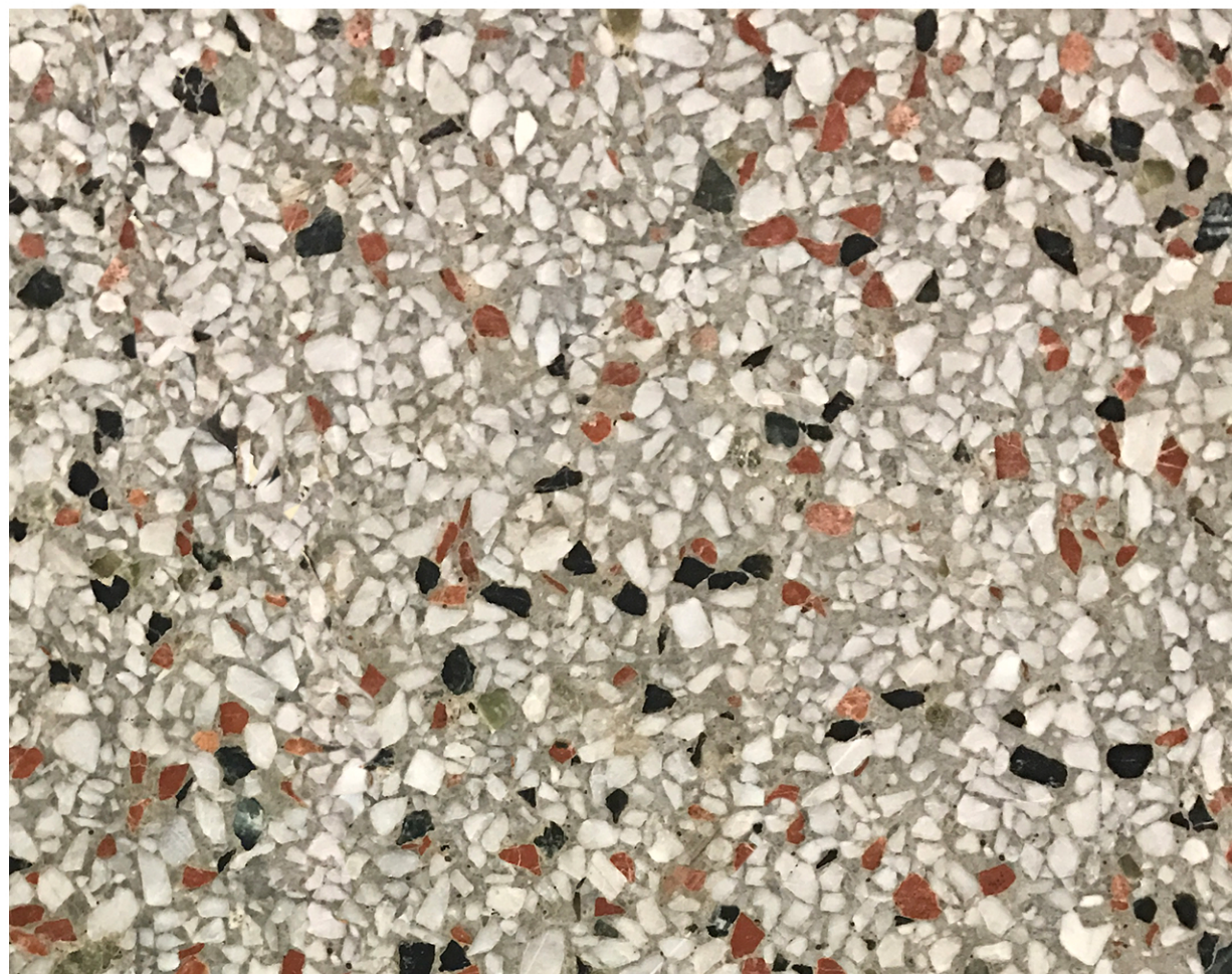
STAIR ONE (21): EXISTING TERRAZZO, NEW TO MATCH
