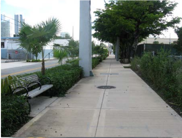
Miami River Greenway on SW 3 Avenue
