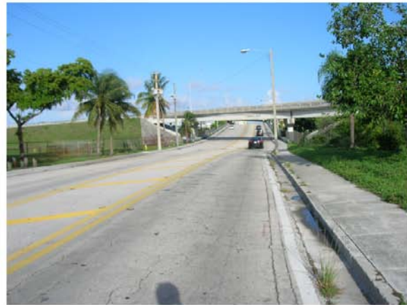
NW 14th Street is an east-west link to the Civic Center.
