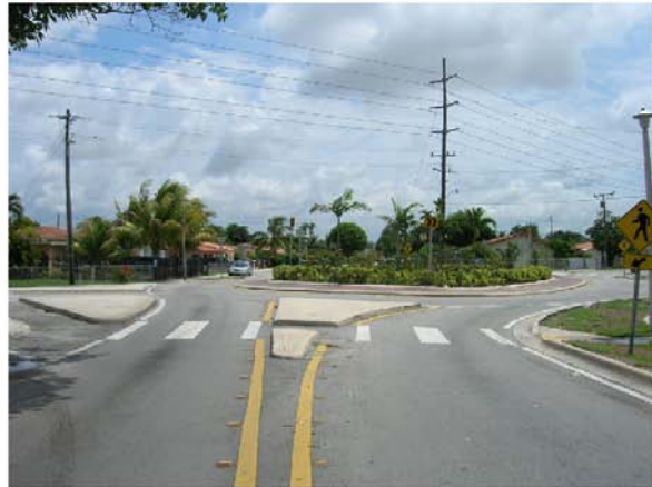
A traffic circle at SW 4th Street and Tamiami Boulevard improves safety.
